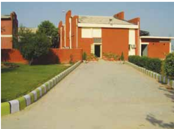
COOLSWAY Structure Plant and proposed PEB Plant at Sikandrabad, UP
