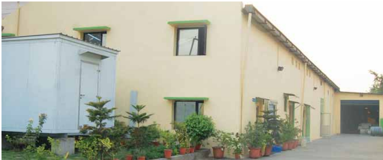
COOLSWAY PUF Plant at Ghaziabad
