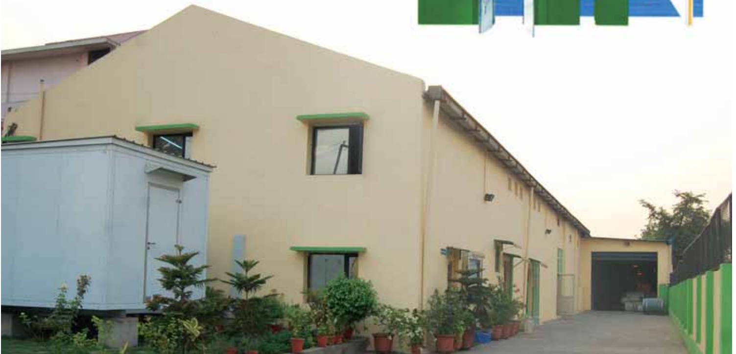
COOLSWAY Plant at Ghaziabad
